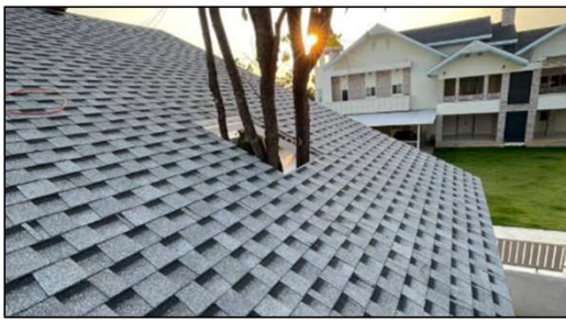
SHINGLE ROOF GREY COLOR WITH MEMBRANE AND OSB BOARD
