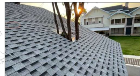
SHINGLE ROOF GREY COLOR WITH MEMBRANE AND OSB BOARD
